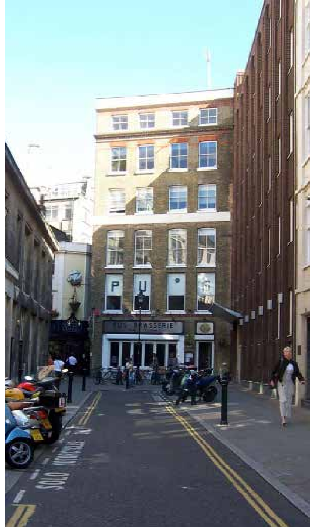
3. View of 10 Gate Street from 6 Gate Street.
