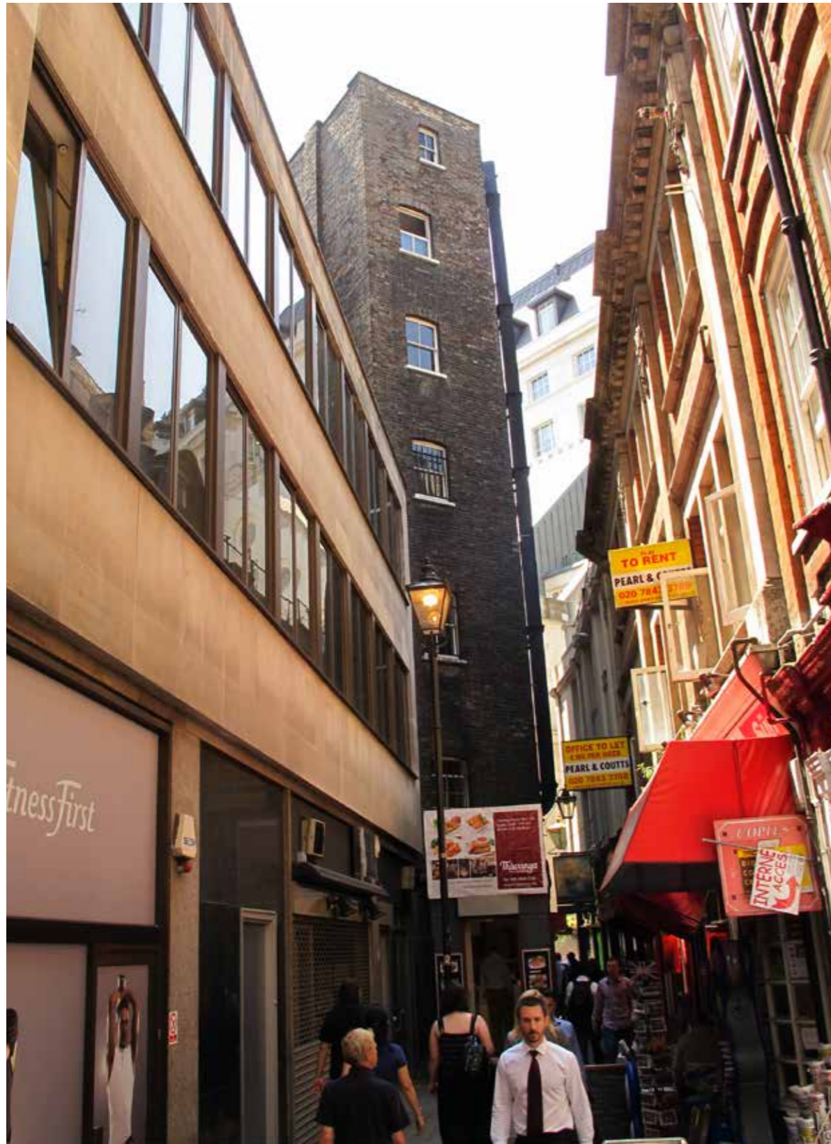
Existing north facade to Little Turnstile Street.
