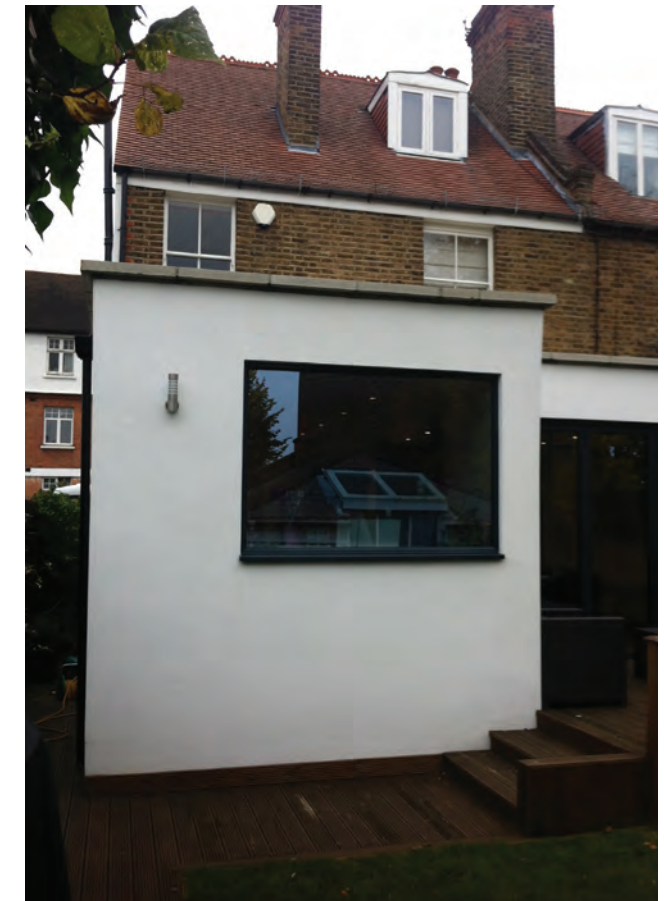
Existing Rear Extension
