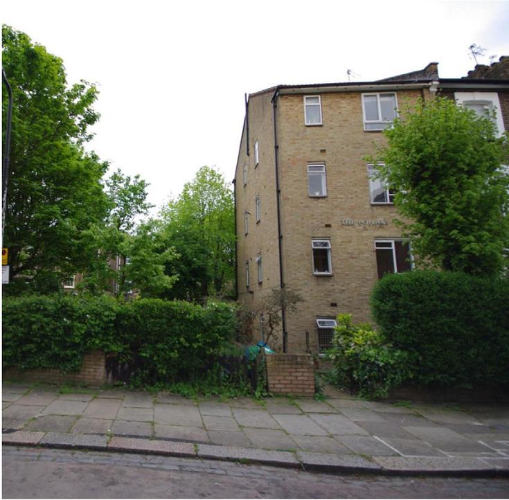
The west facade of The Poplars faces Montpelier Grove and follows the rhythm of the terrace in its scale and in the arrangement of windows to living spaces. The block is clad with yellow bricks to match the rest of the terrace, though the bricks of the Victorian terrace have weathered and stained to a darker colour.
