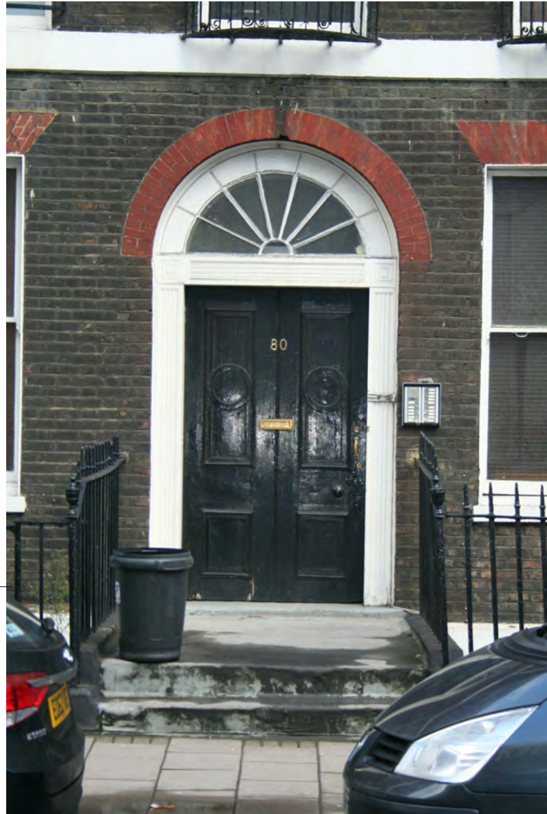
Exterior front door
