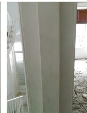
DF-01 View of door frame on 1st floor landing
