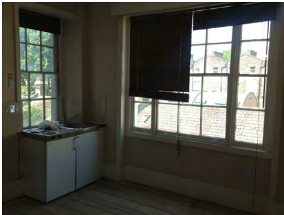
Window WF-04 and rear 1st floor side window
