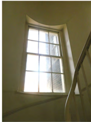
Dado railing profile 1 on stairs
