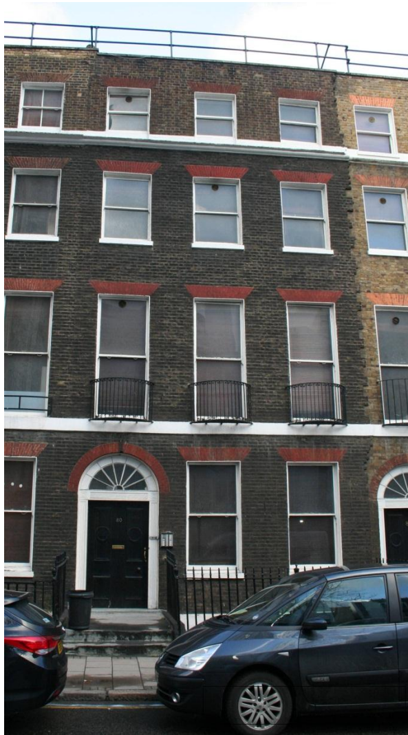
Fig 1: Front façade of the building with original box sash windows
