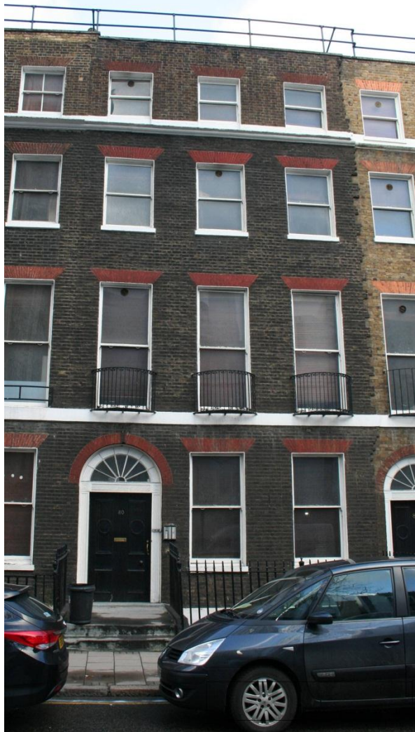
Fig 1: Front façade of the building with original box sash windows
