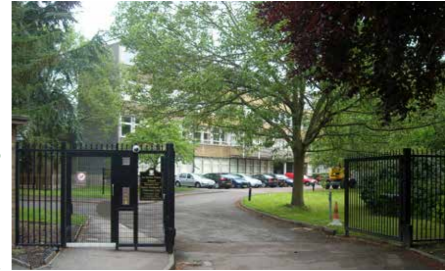
photo of existing site access
