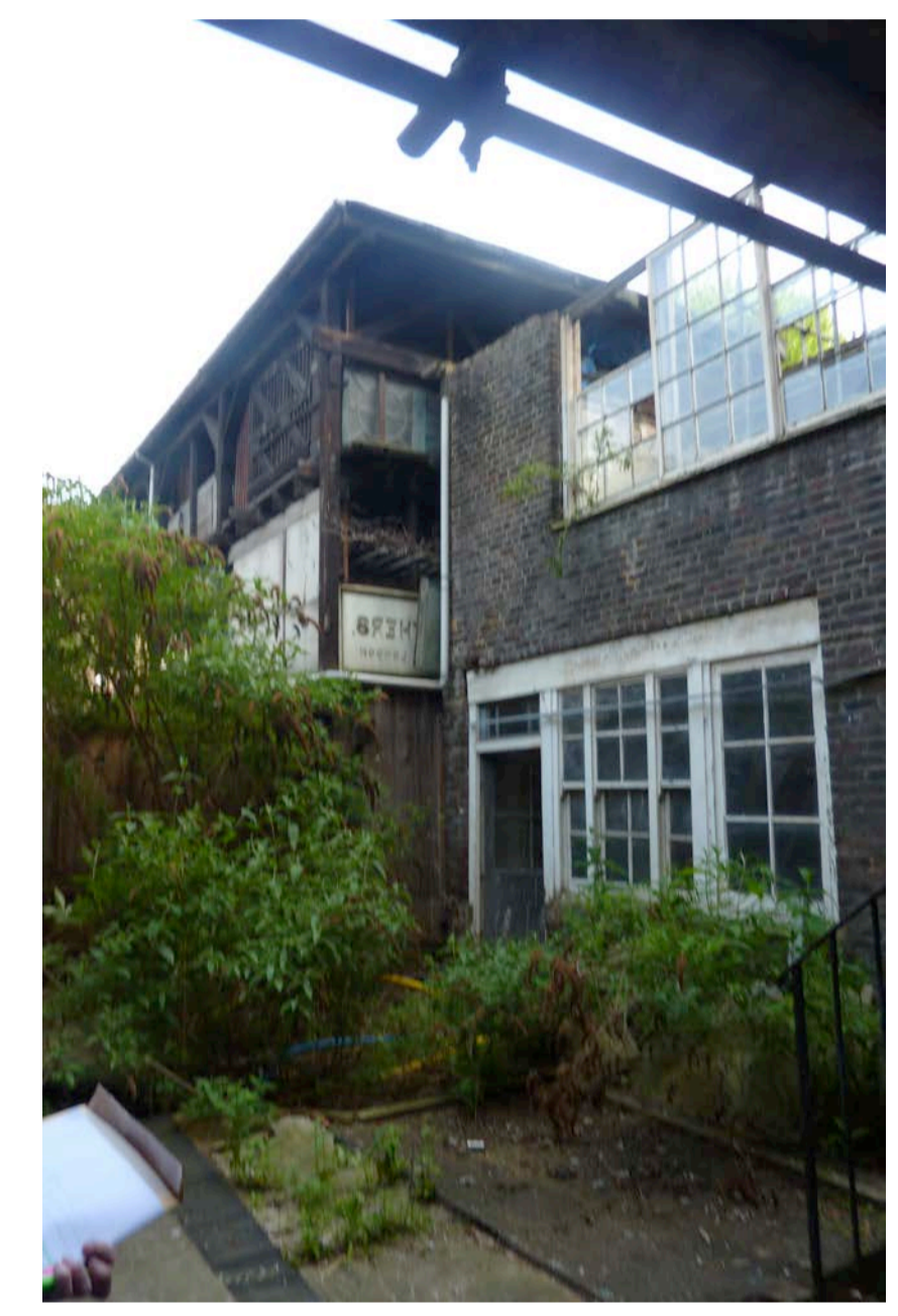
DOOR HEIGHT AND TOP OF WINDOW LEVELS TO MATCH EXISTING AS SHOWN
