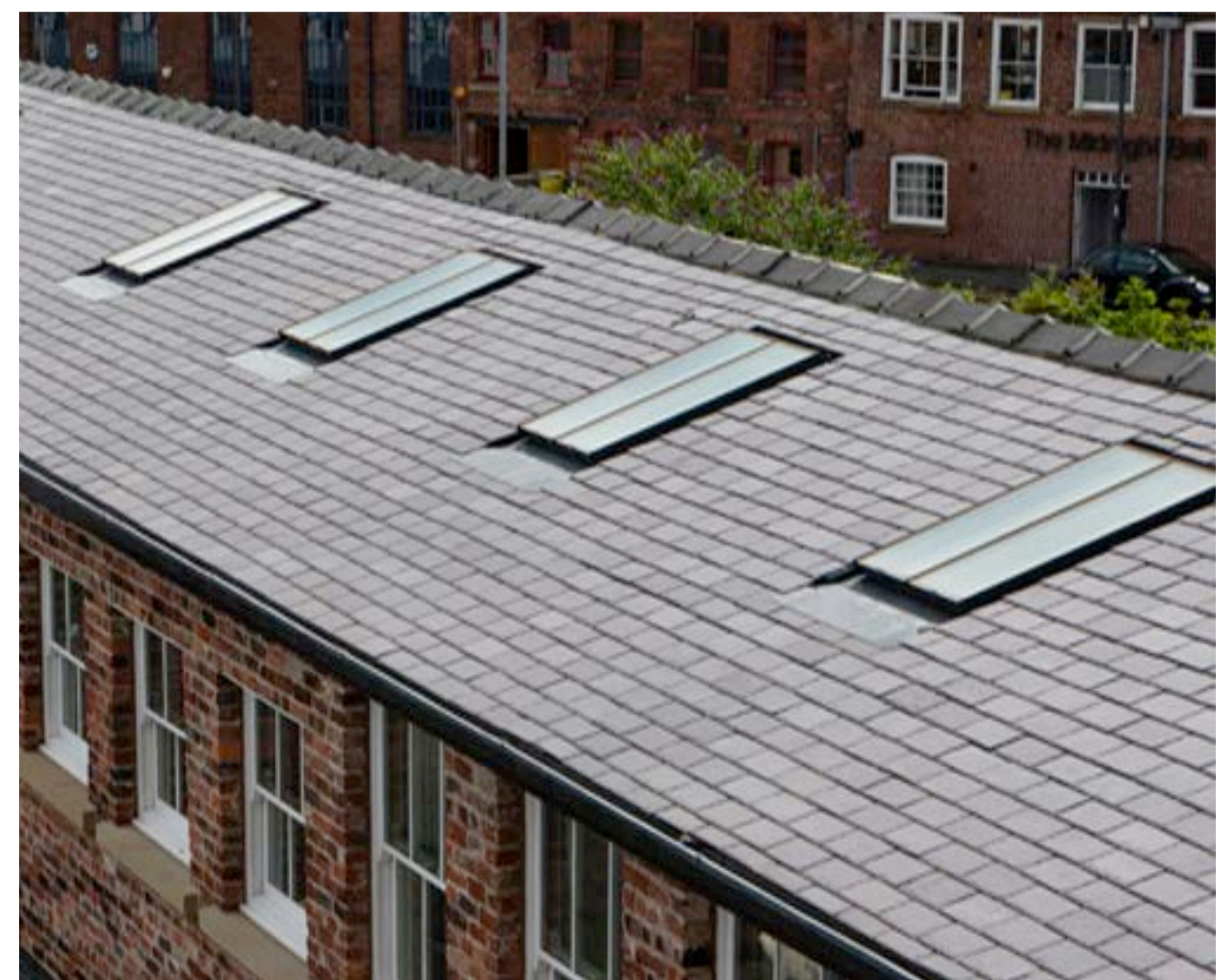
PHOTOGRAPH OF PROPOSED ROOFLIGHTS TO BE POSITIONED INLINE WITH ROOF SLATE LINE AT SAME LEVEL AS EXISTING
