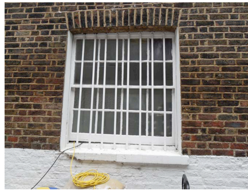
TWO MATCHING EXISTING WINDOWS TO BE RECREATED AS SHOWN IN SIZE, TYPE & LOCATION
