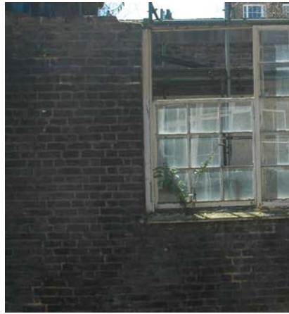
EXISTING BRICKWORK MULTI STOCK RED BRICK FLEMISH BOND
