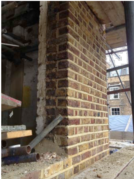
ORIGINAL BRICKWORK: MULTI STOCK YELLOW BRICK ENGLISH BOND
