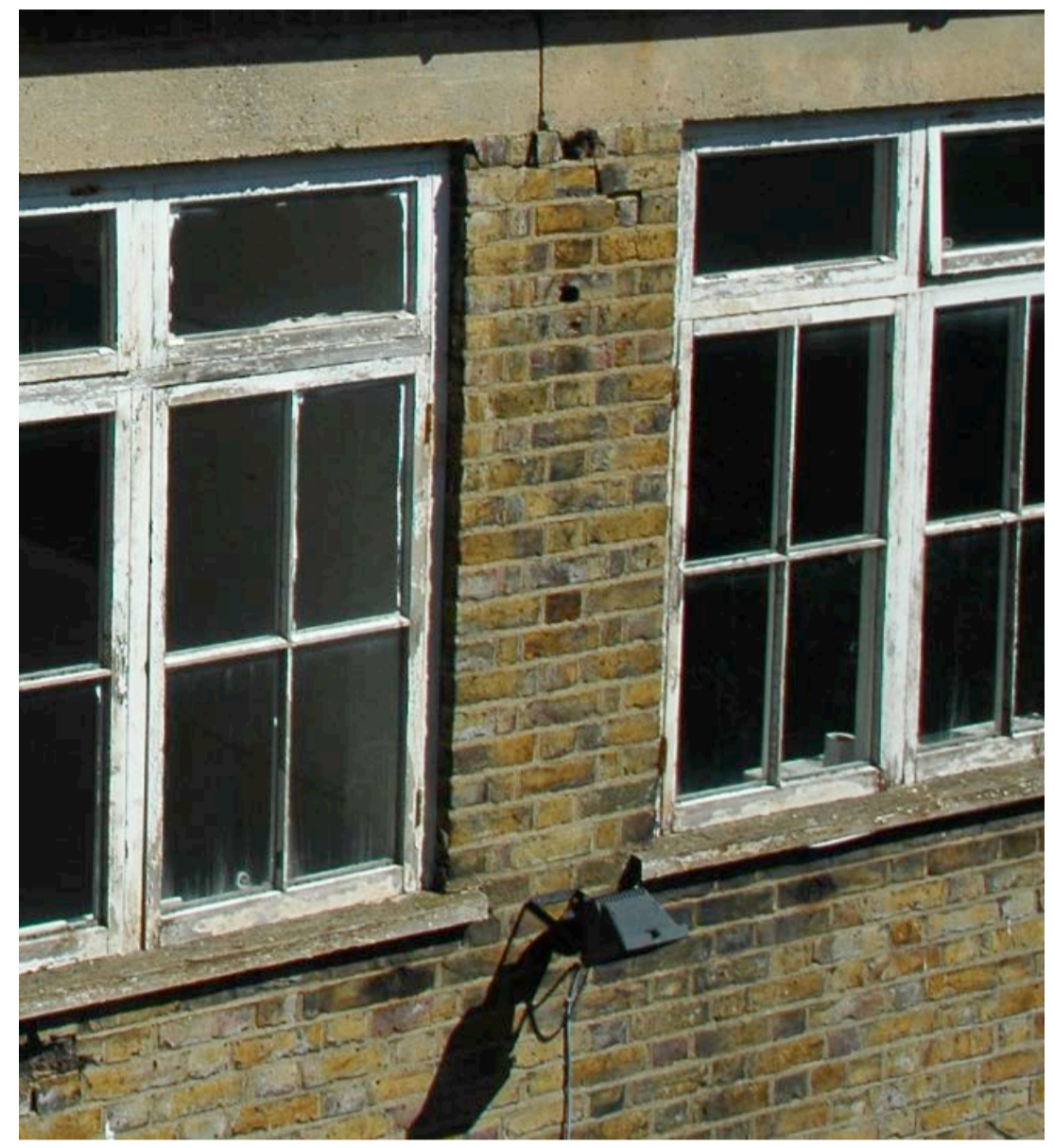
BRICK PIERS BETWEEN WINDOWS AS EXISTING
