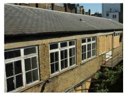
EXISTING - SHOWING FLEMISH BOND AND CONCRETE LINTELS TO BE REINSTATED
