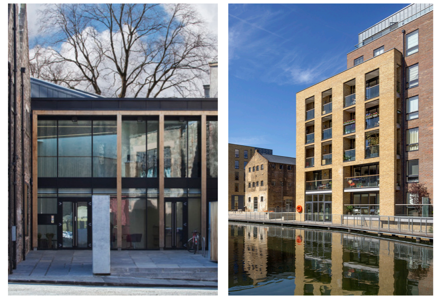
Precedents above: Left: Greyfriars Community Project (Gareth Hoskins Architects) showing use of framing in front of curtain walling giving a light and transparent appearance Right: Kingsland Wharves (TM Architects) showing use of regular grid of openings with inset balconies behind
