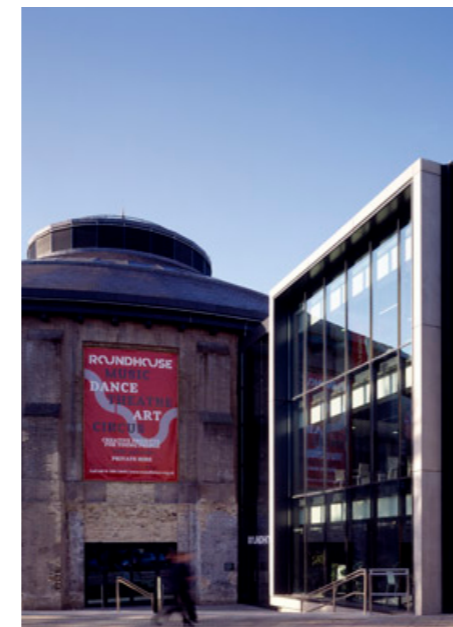
Photograph of the completed extension from the exterior
