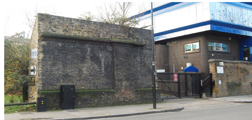
Remaining section of original retaining wall at east end of site
