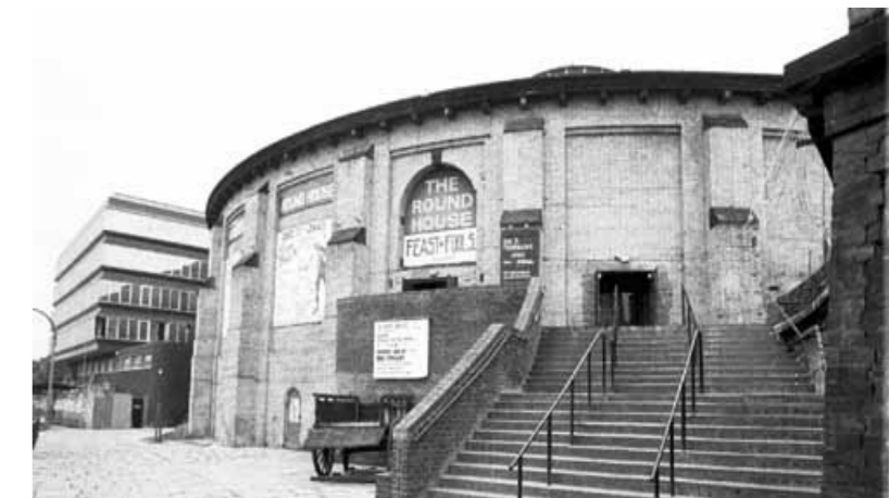
Photograph of the Roundhouse c 1974 (with the new 100 Chalk Farm Road in the background)
