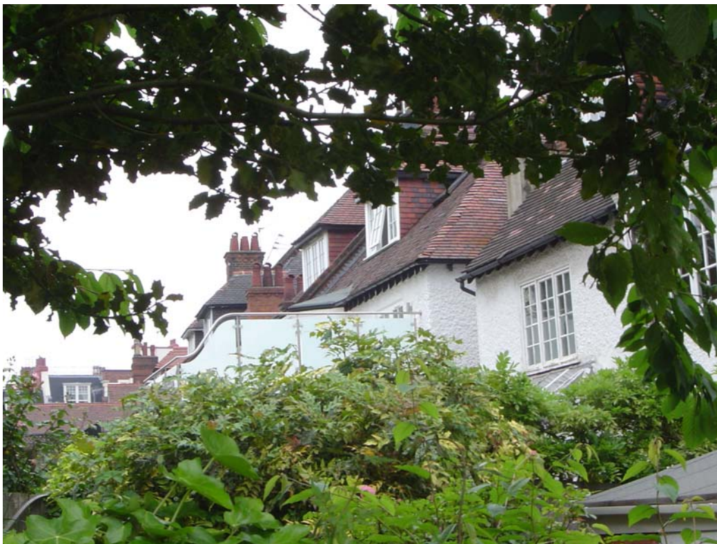
PLATE B: VIEW OF TERRACE OF THE NEIGHBOURING PROPERTY (NO.39 CREDITON HILL)
