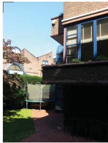
View north west (South Elevation)
