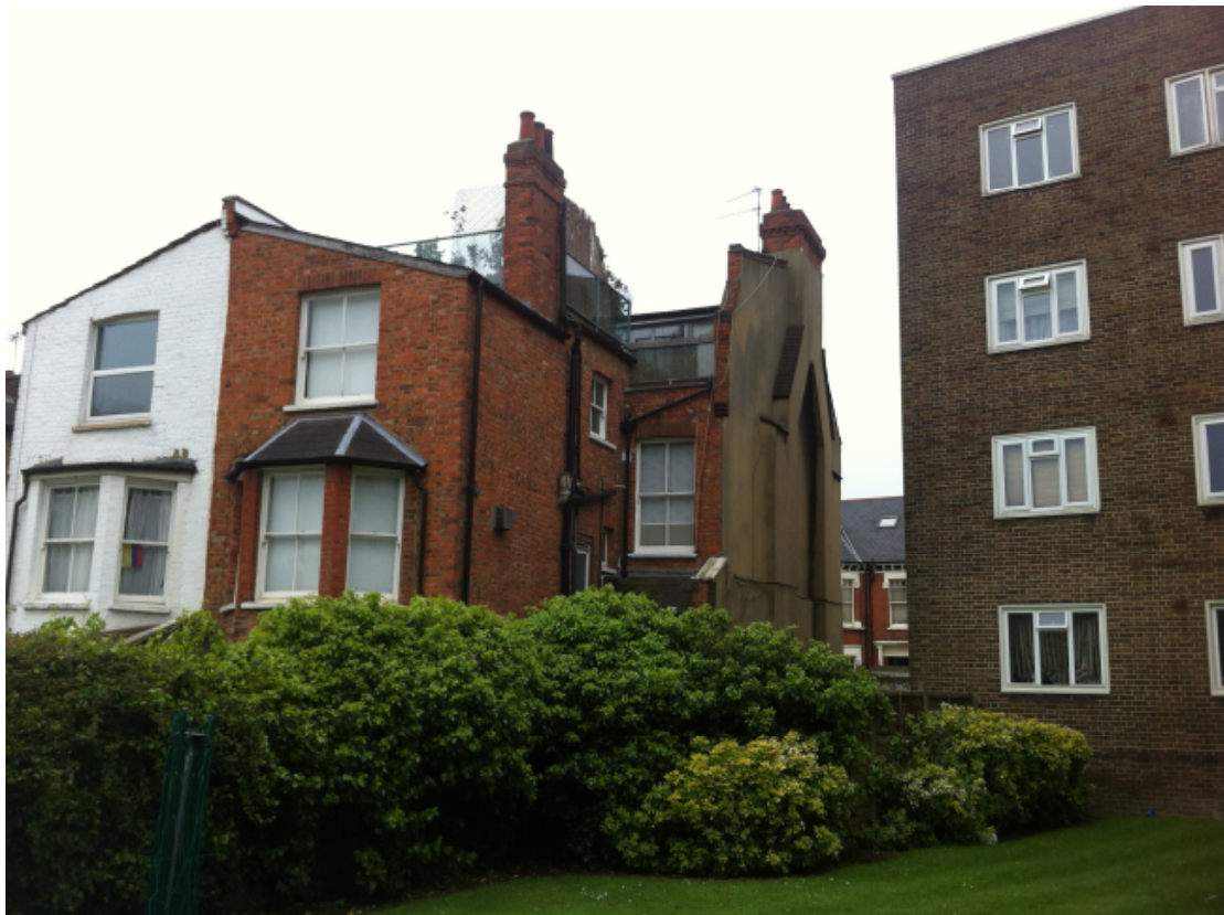
Rear of 31 Holmdale Road with the site between this and 33-39.
