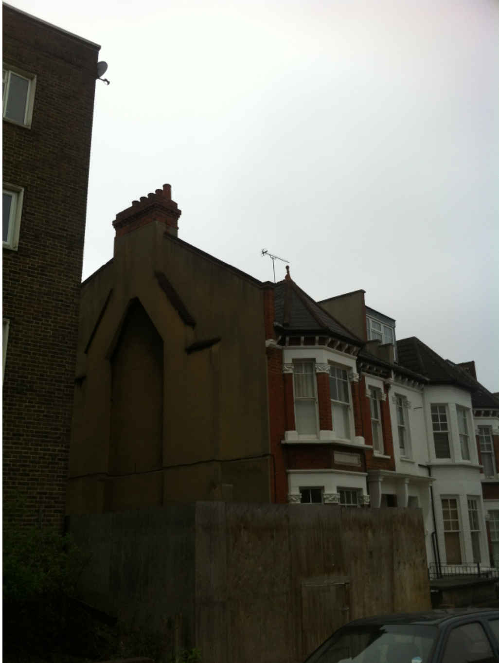
View of site from in front of 33-39 Holmdale Road (to the north)
