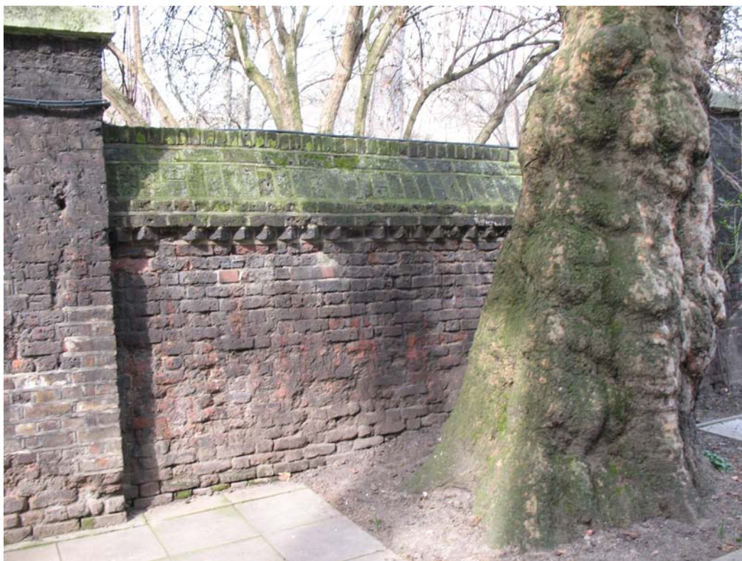
Photograph 21: Wall panel 25 general condition
