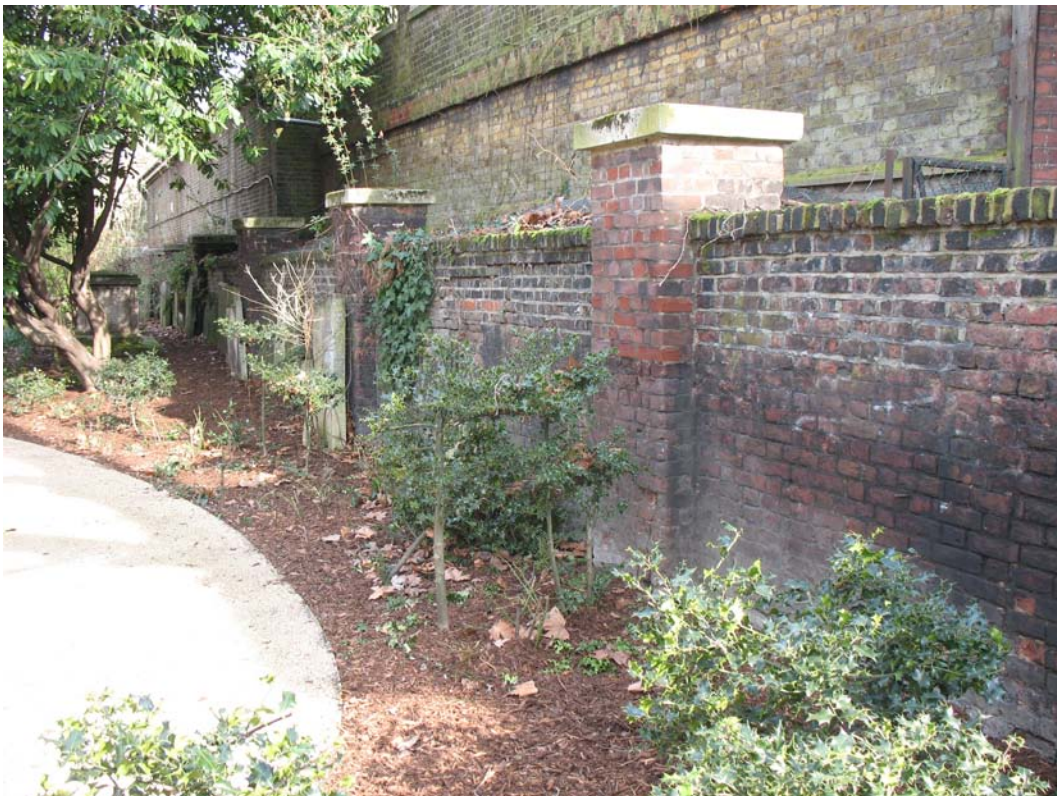
Photograph 2: Typical elevation of north elevation
