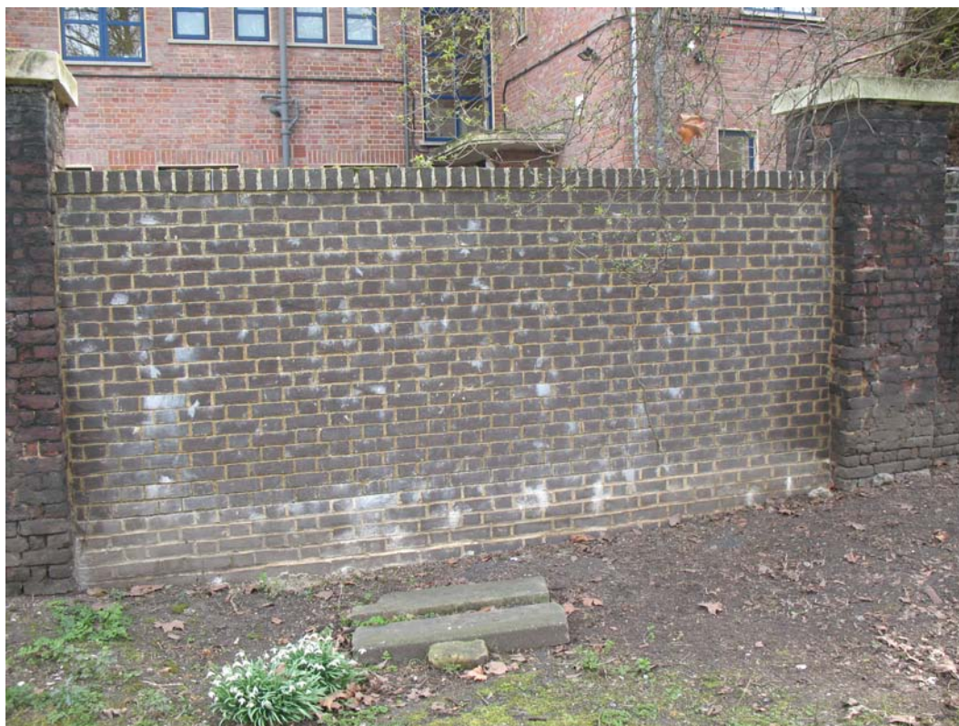
Photograph 11: Reconstructed wall panel 24
