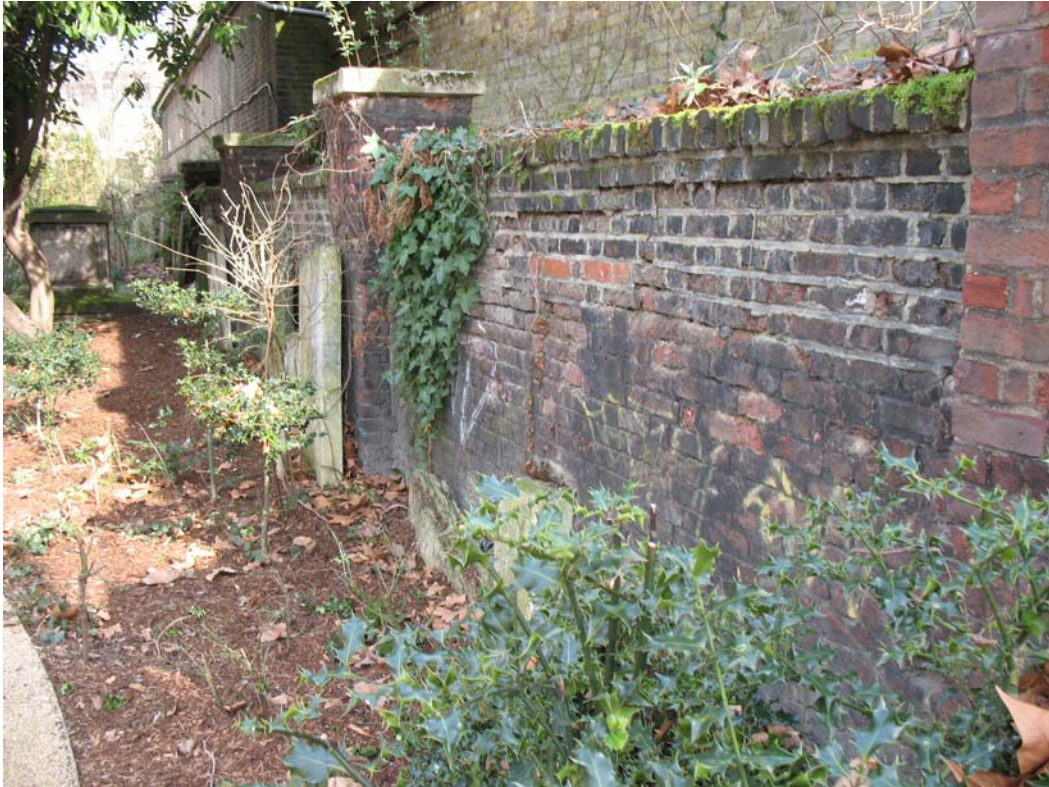
Photograph 9: Wall panel 16 showing horizontal movement in top courses
