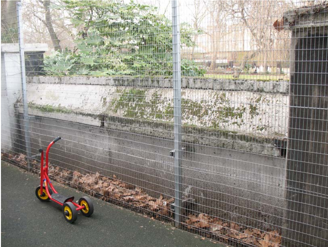
Photograph 15: Panel 6 with wire fencing attached to wall
