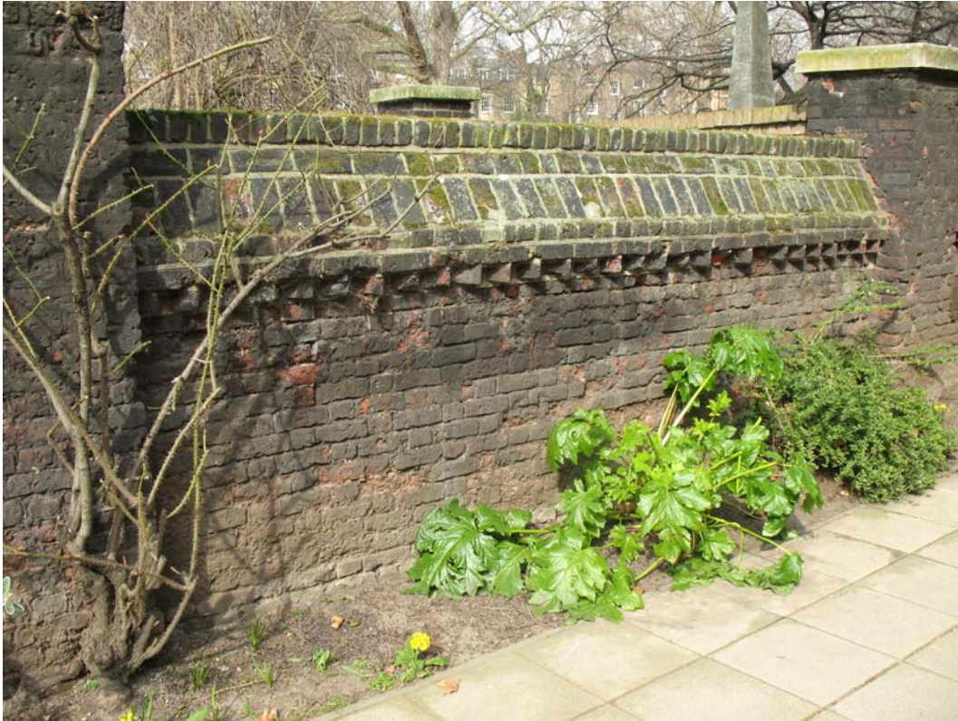
Photograph 1: Typical elevation of south elevation showing piers and dog tooth course
