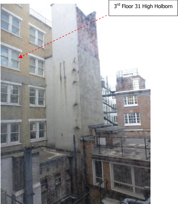
Photograph 3 - Nearest residential receptor
