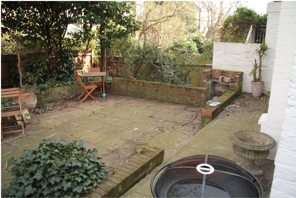
Extension Built at 5. Denning Road
