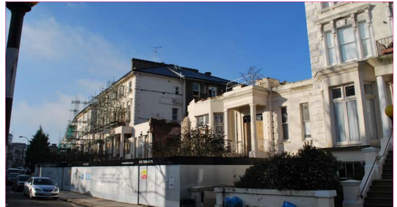
Looking south-west along Belsize Park
