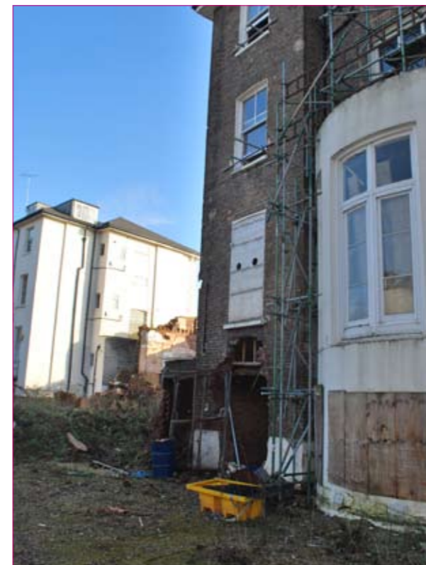
The rear of 44 Belsize Park, looking north with 41 in the distance
