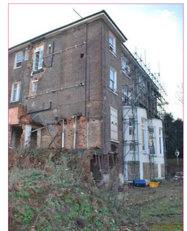
The rear of 44-45 Belsize Park, looking south
