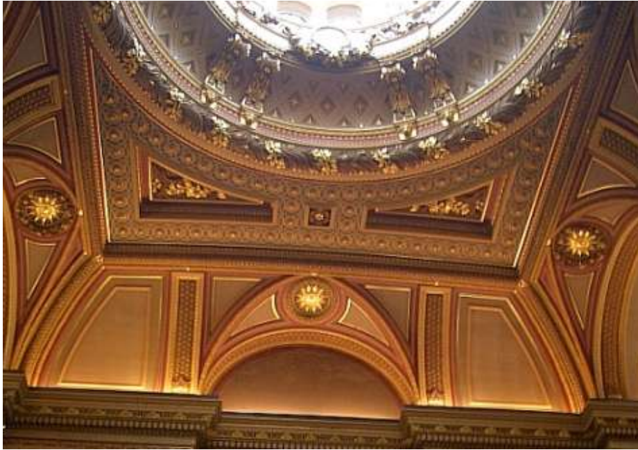
Illustration 7.07 Layered domed ceiling over the main staircase in the Fitzwilliam Museum, Cambridge, designed by Geroge Basevi. Basevi uses the diagrid form for both structure and decoration, most effectively in the upper section, creating a visual and spatial dynamic to the space
