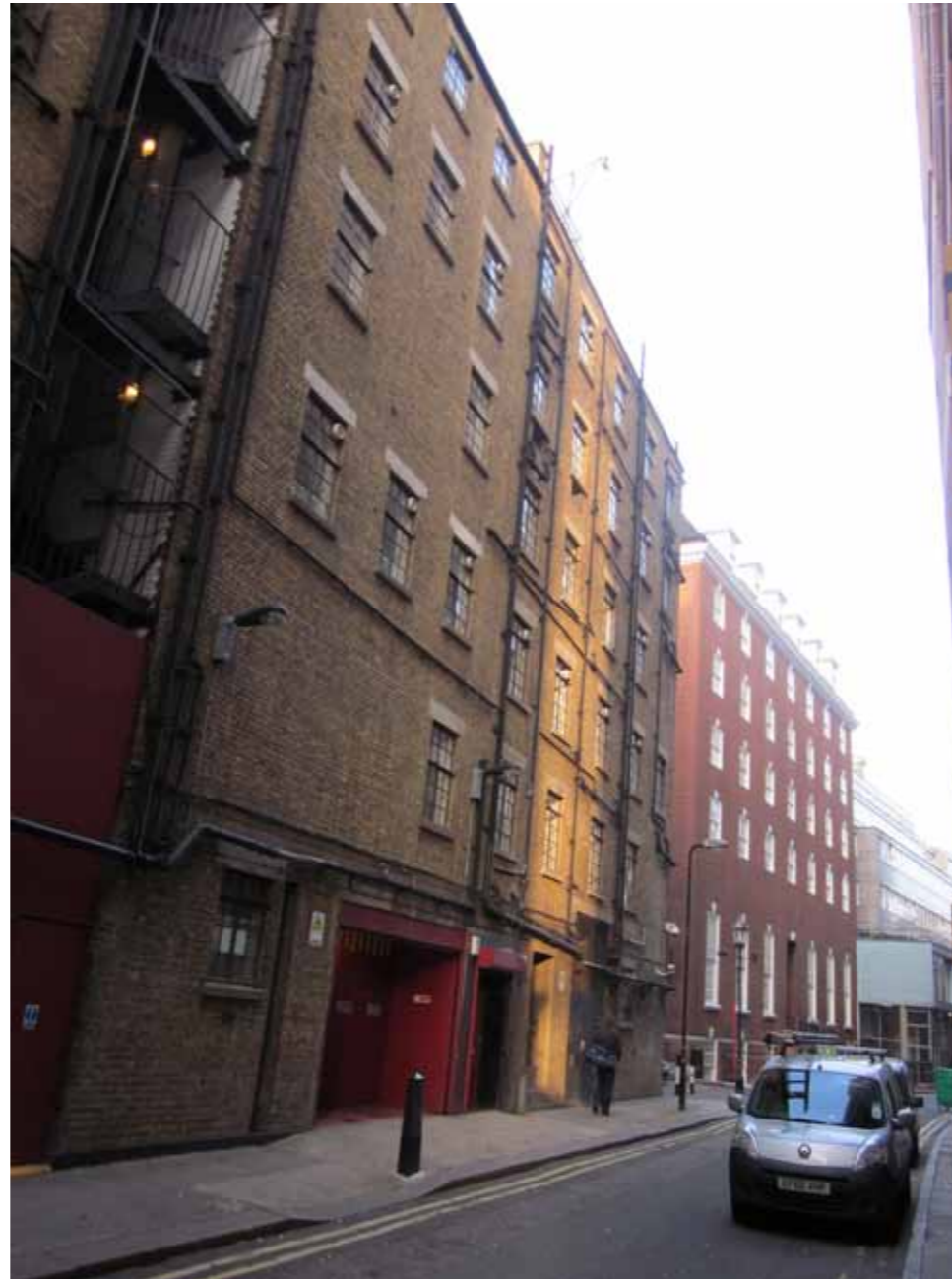
6 View of Rear of Theatre and Bainbridge Street
