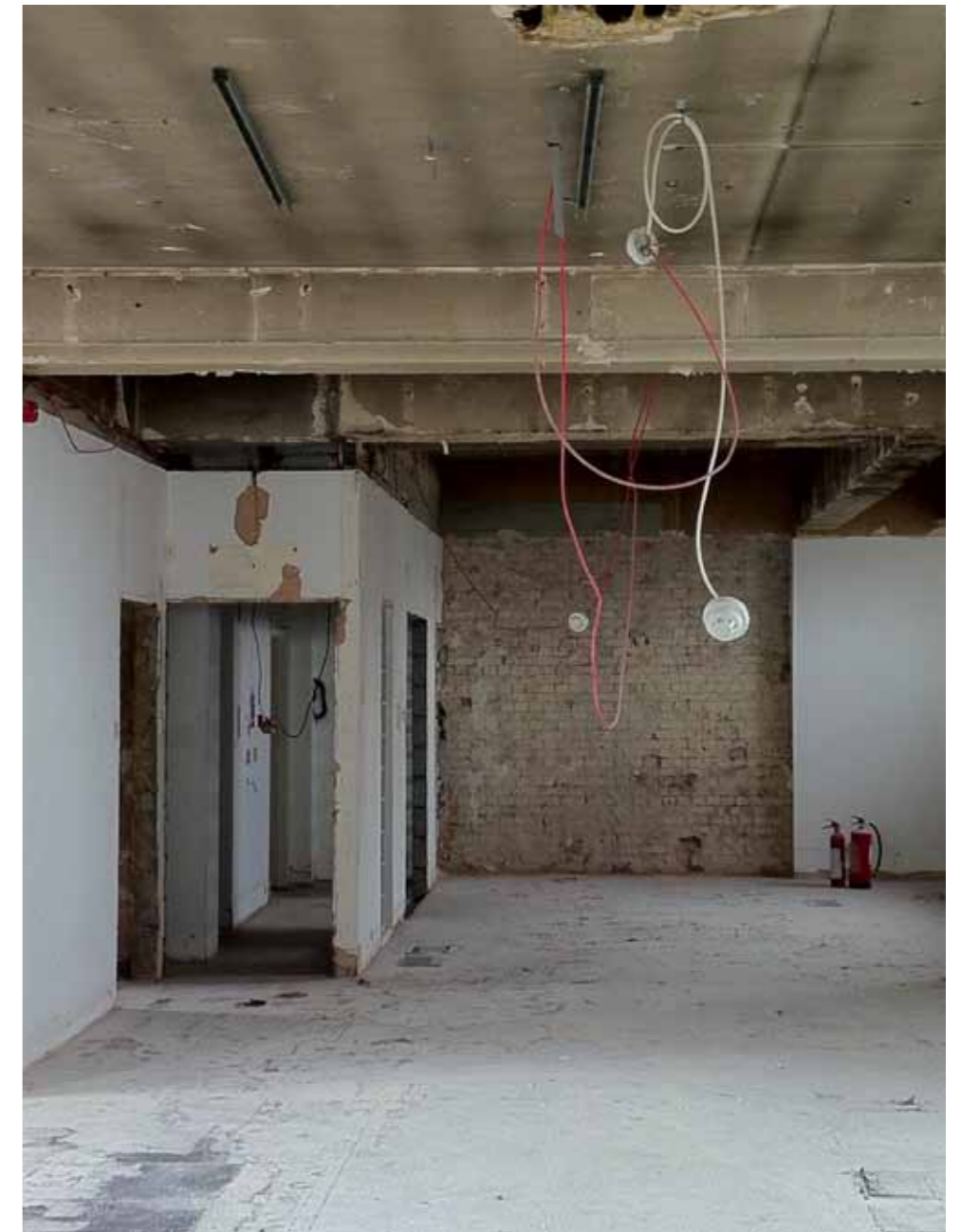
► View of 6th Floor
