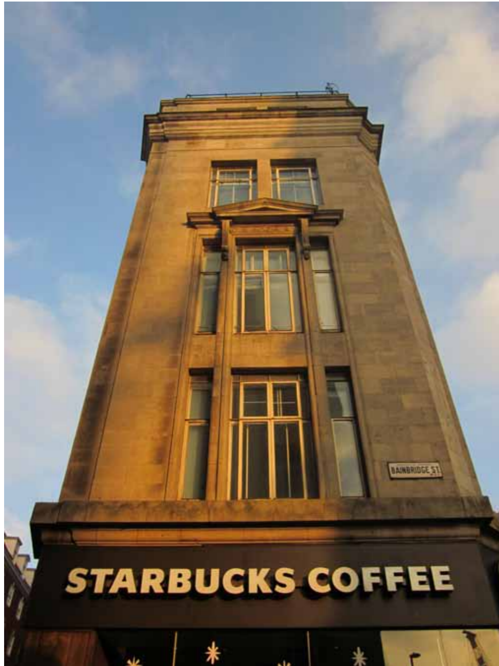
2 Corner of Building Where it Turns into Bainbridge Street.
