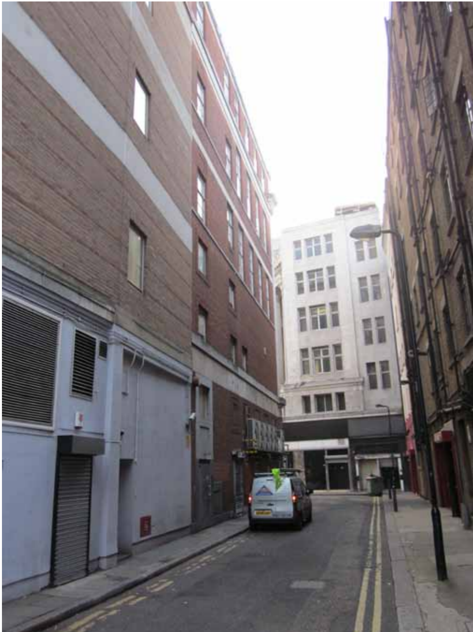
5 Bainbridge Street Rear Facade.
