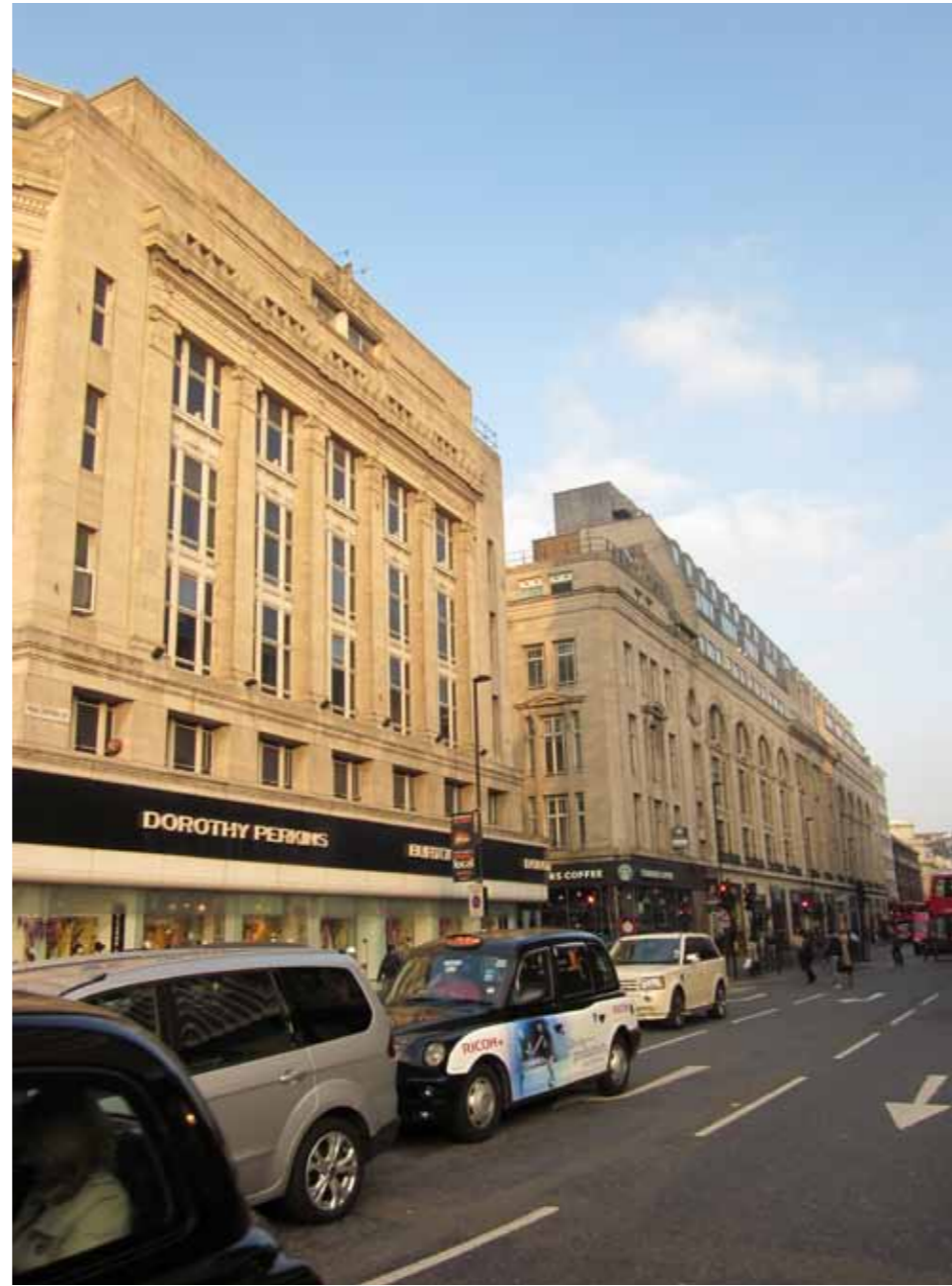
3 View of existing building from Tottenham Court Road and New Oxford Street junction, party wall and stepped height with neighbouring building visible
