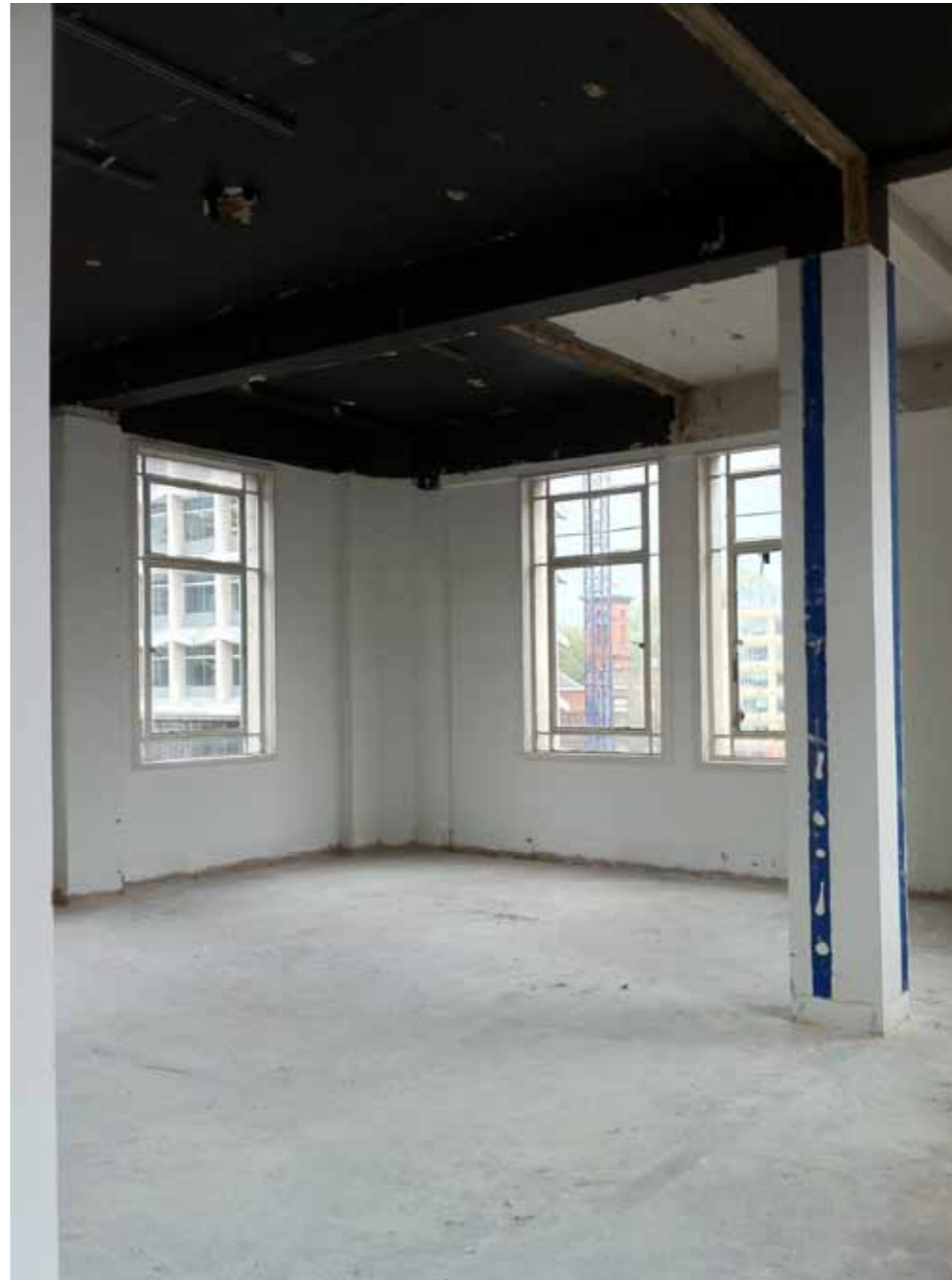
► View of 5th Floor
