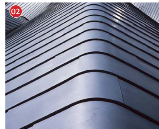
Zinc Roof Cladding
