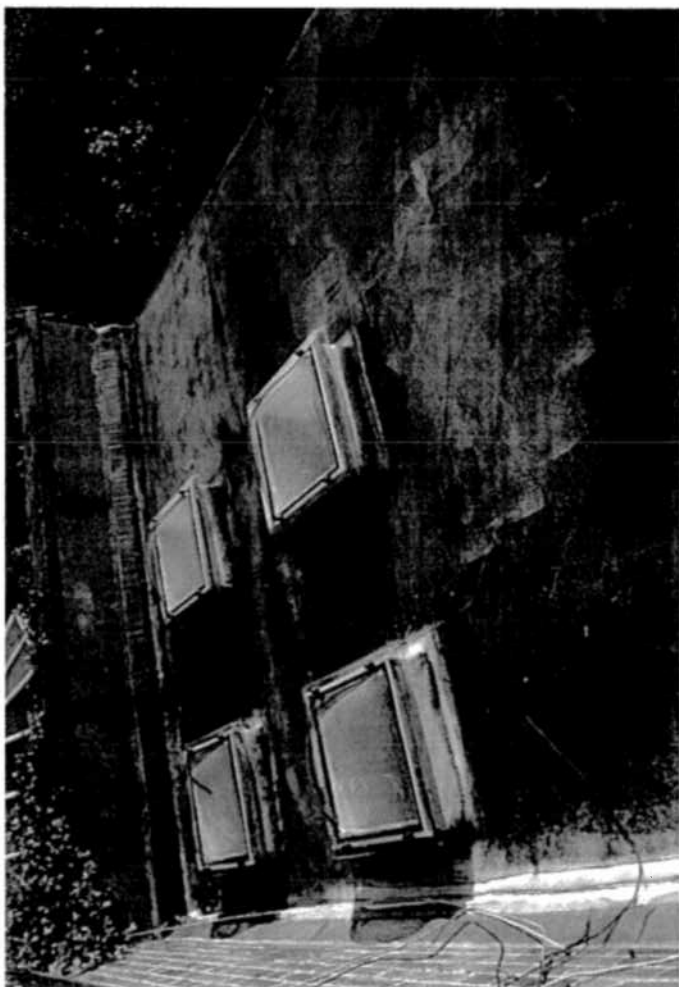
Existing gas roof
