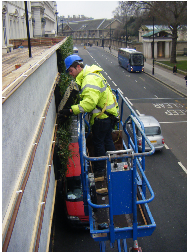
PCND Driplines installed @ Buckingham Gate
