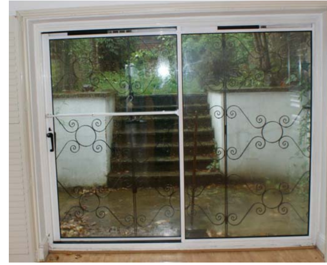
17-03 Existing Ground Floor Sliding Door
