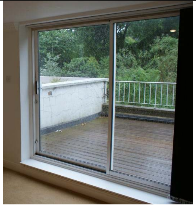
17-05 Existing First Floor Sliding Door
