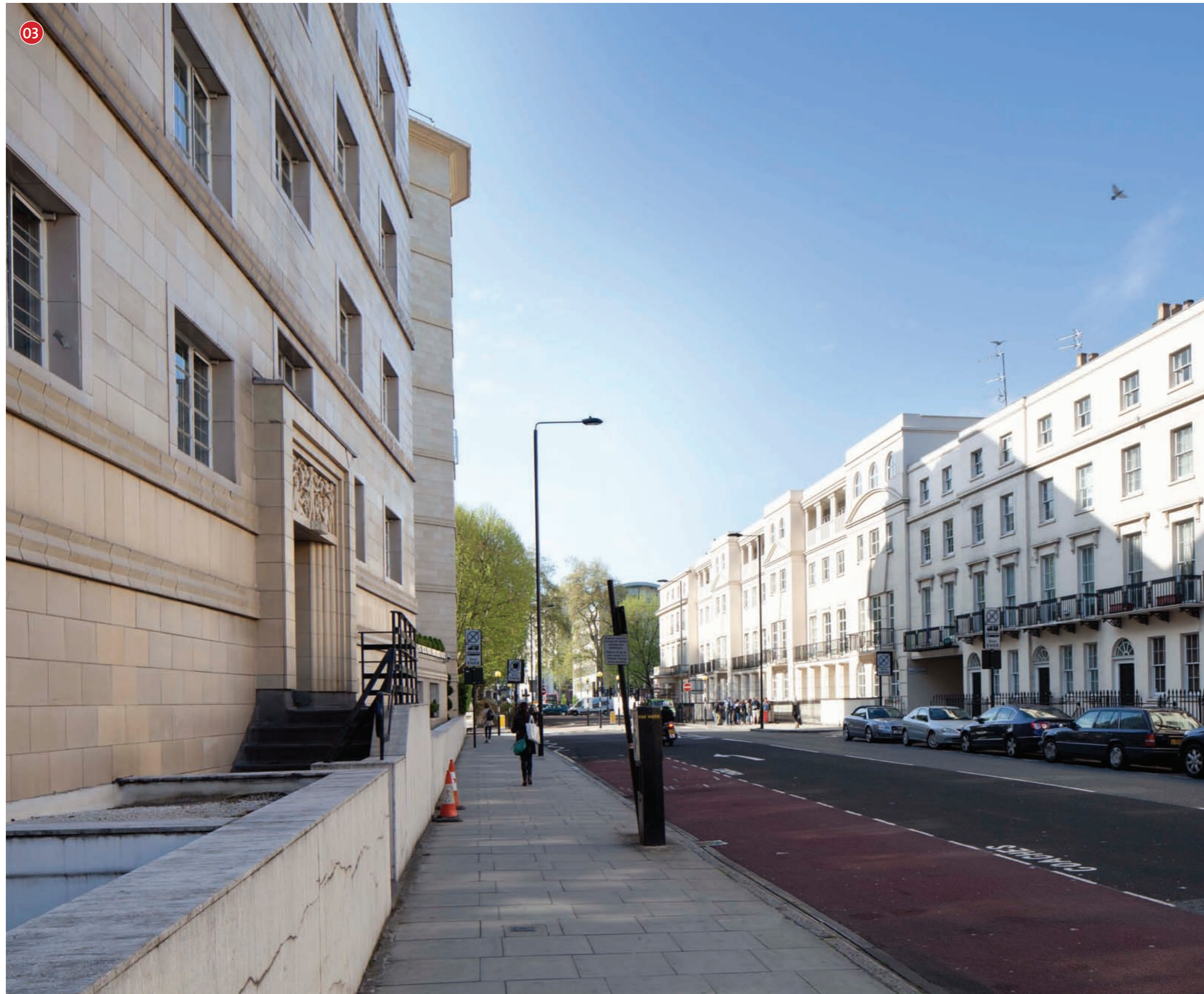
Existing View from Albany Street Looking South
