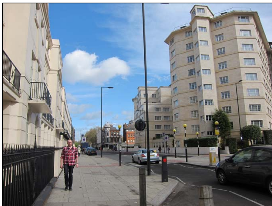
Plate 10: View facing north along Albany Street with 1-9 Albany Street to the left of the photograph and the contrasting form of the White House to the right.
