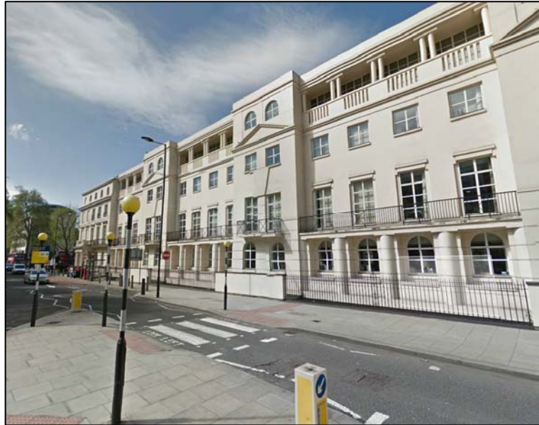
Plate 4: Modern view of 1-9 Albany Street facing southwest. The elevation is a modern interpretation of the Nash-style with poor architectural detailing, inappropriate proportions and poor use of motifs.
