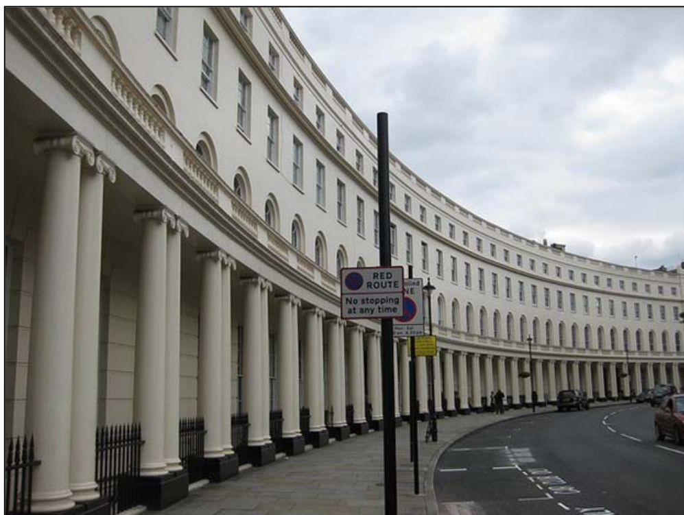
Plate 12: Park Crescent facing south, illustrating the rhythm of coupled Ionic columns across the ground floor.
