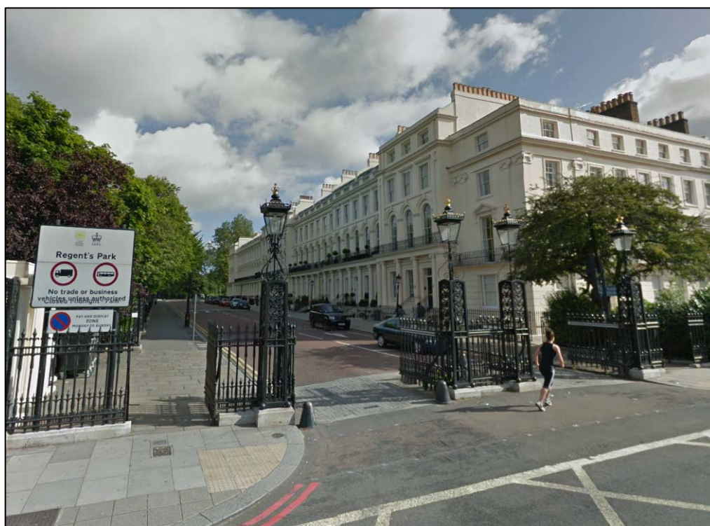
Plate 6: 13-24 Park Square East facing north, with 1-3 Albany Terrace. These Nash terraces date to 1823-5 and is formed of 12 houses.
