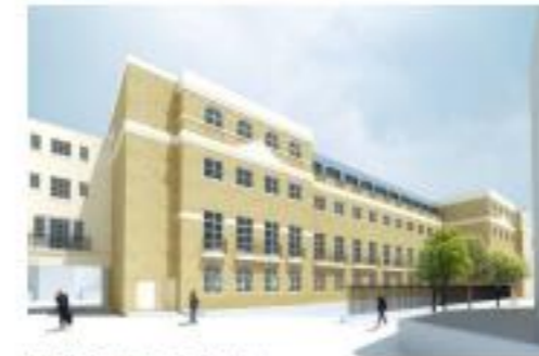
Existing View Looking South East into Peto Place
