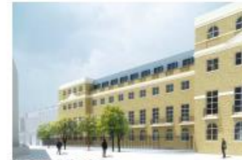
Existing View Looking North East into Peto Place
