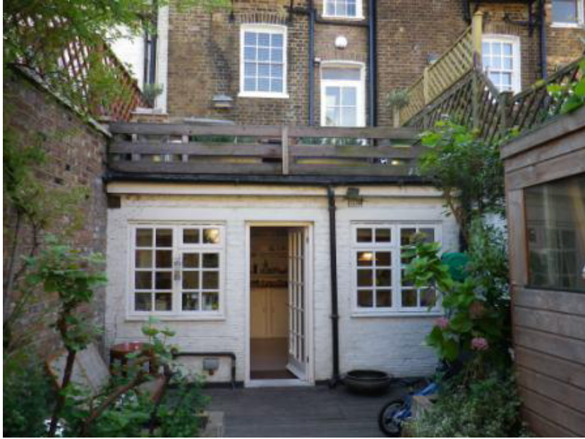
Rear elevation 21 Hartland Road
