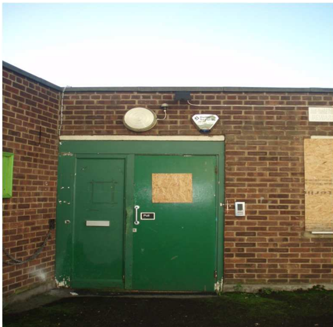
Image 11: Secure Entrance to Disused Section of Greenwood Place
