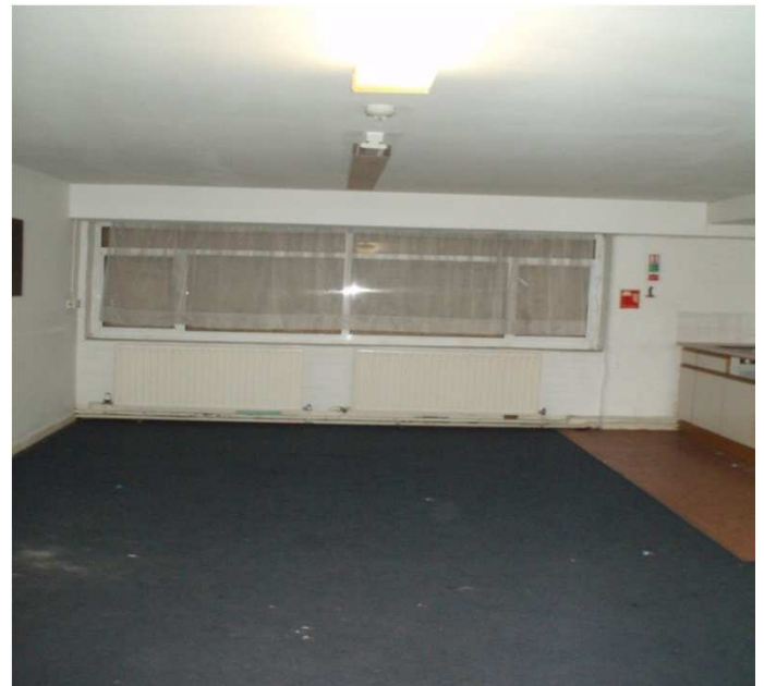
Image 12: A Room within the Disused Building
