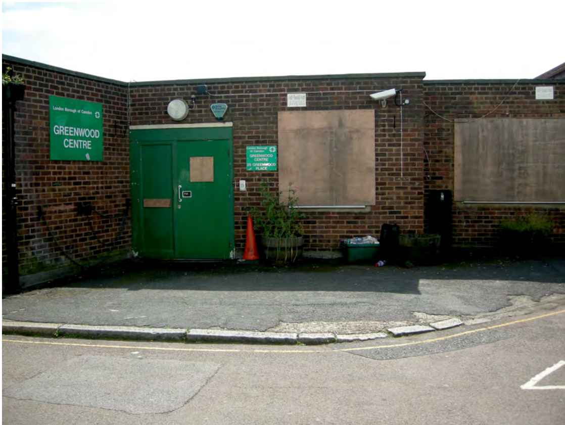
Fig 14 Former Greenwood Day Centre at 25 Greenwood Place, looking south-west (MOLA, 2010)
