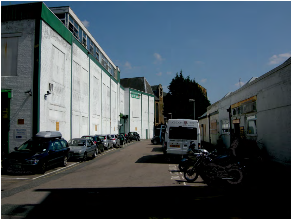
Fig 12 The central stretch of Greenwood Place, looking south-east, with A&A Self-storage (19 Greenwood Place) on the left and The Camden Society (37 Greenwood Place) on the right (MOLA, 2010)
