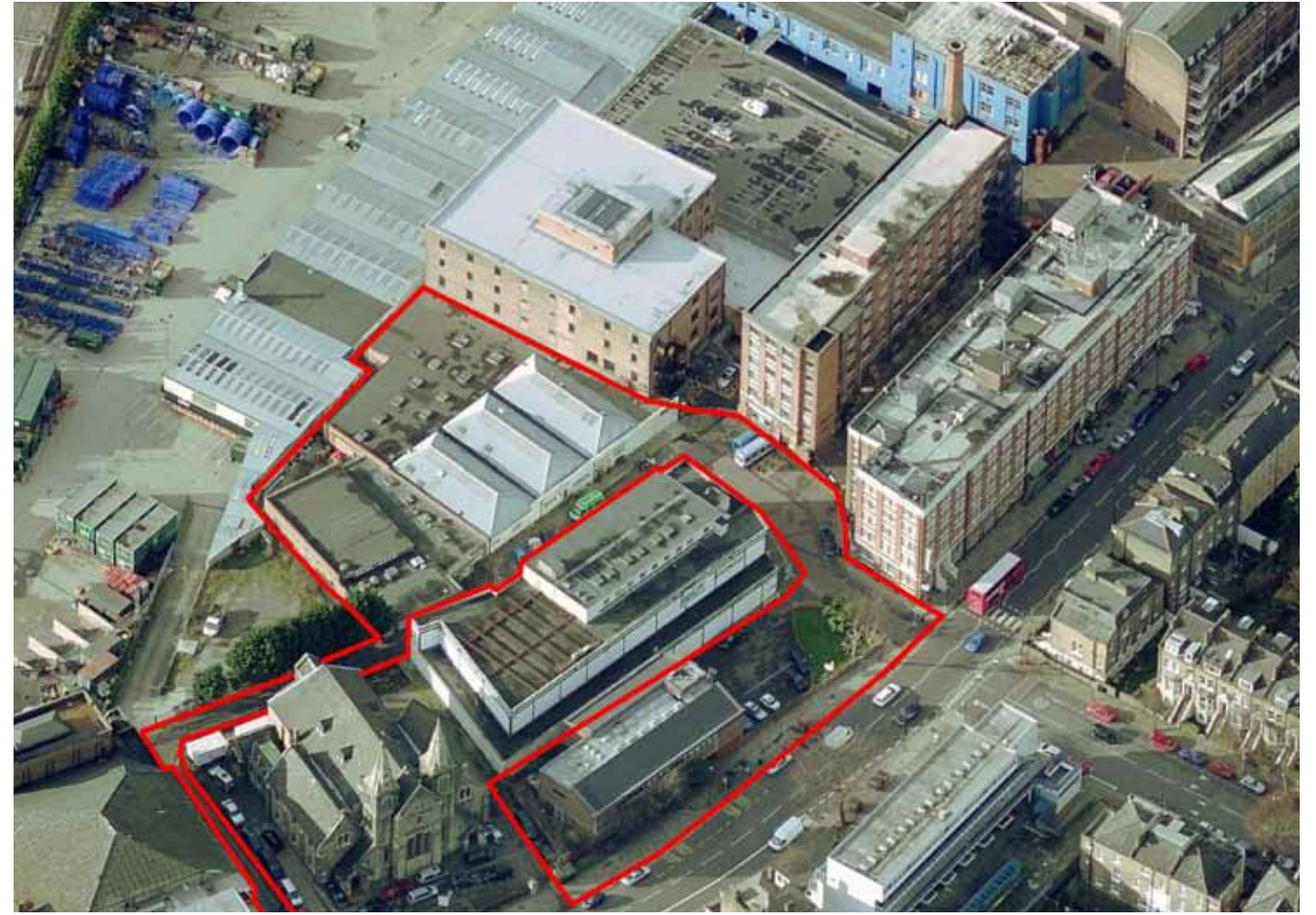
Aerial view looking west
