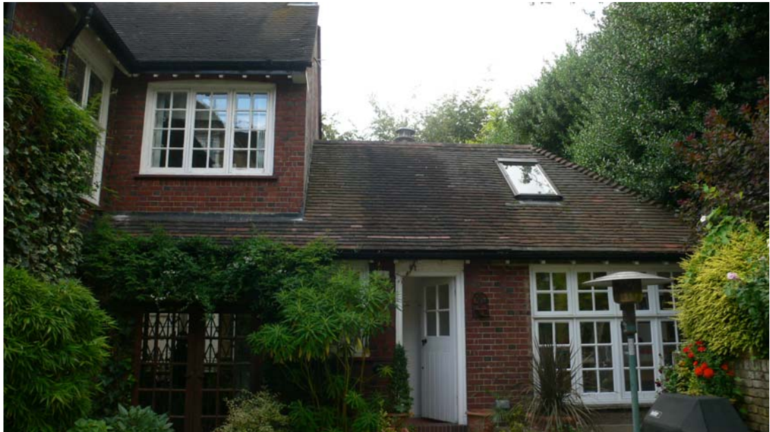
Photo 4 – Rear of house taken from rear garden looking NW.
