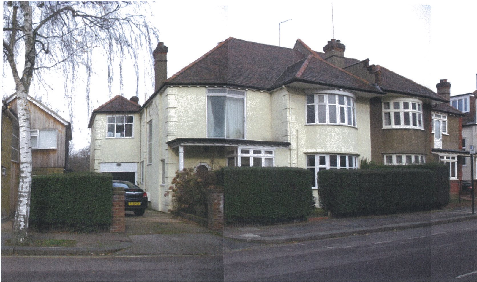
30 Menelik Road - Front Façade
