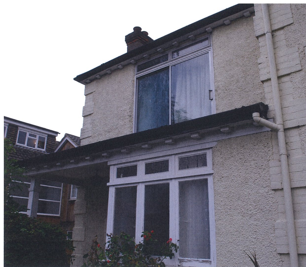
Existing Porch Canopy and Verandah
