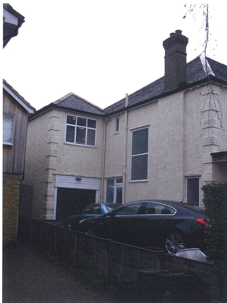
Existing Side Wing with Garage
