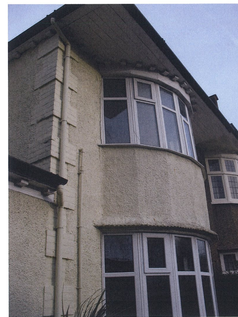
Existing uPVC Bow Window to be Replaced with Traditional Timber Frames
