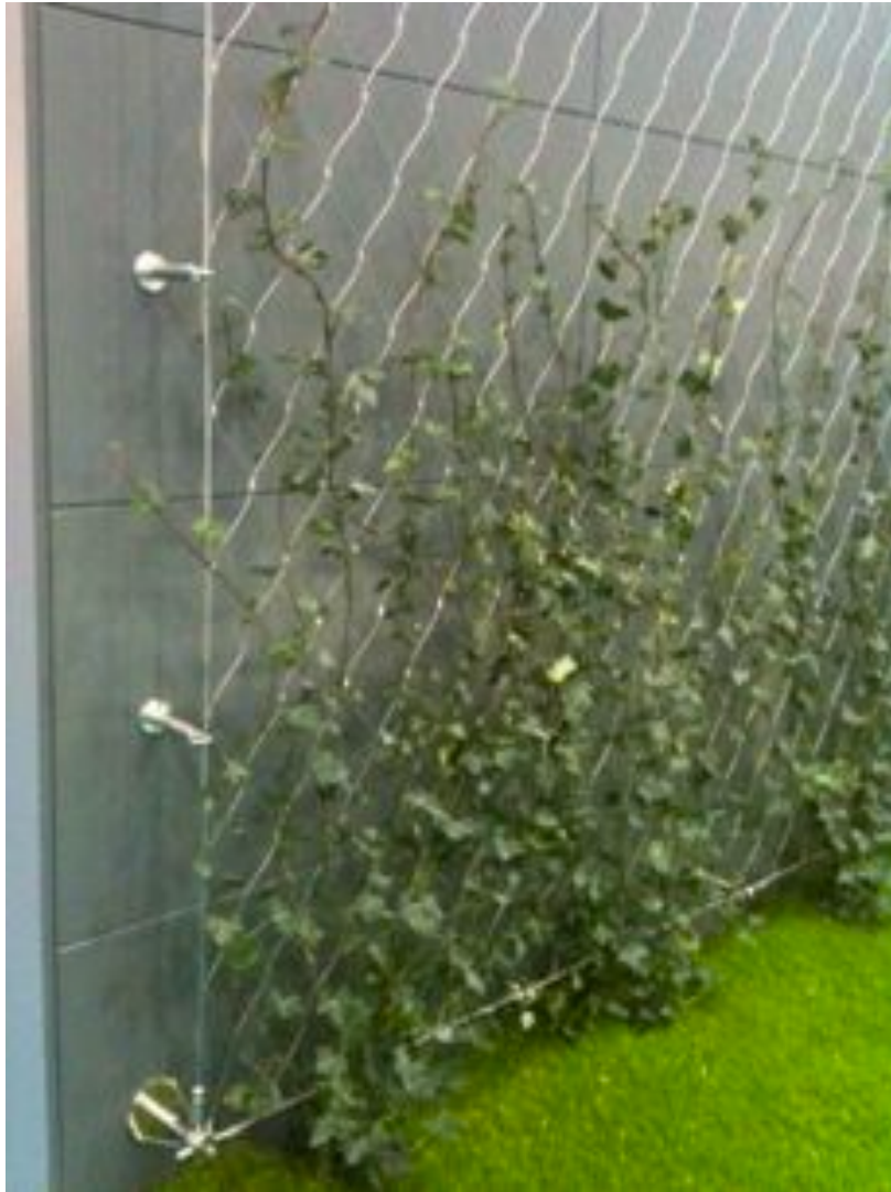
Image above showing tension cabling with climber, Low tech, low maintenance green wall
