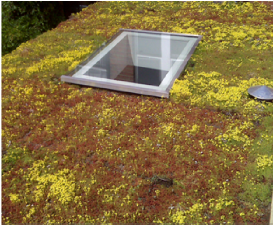
Image of sedum green roof as proposed for the rear and side extension roof tops
