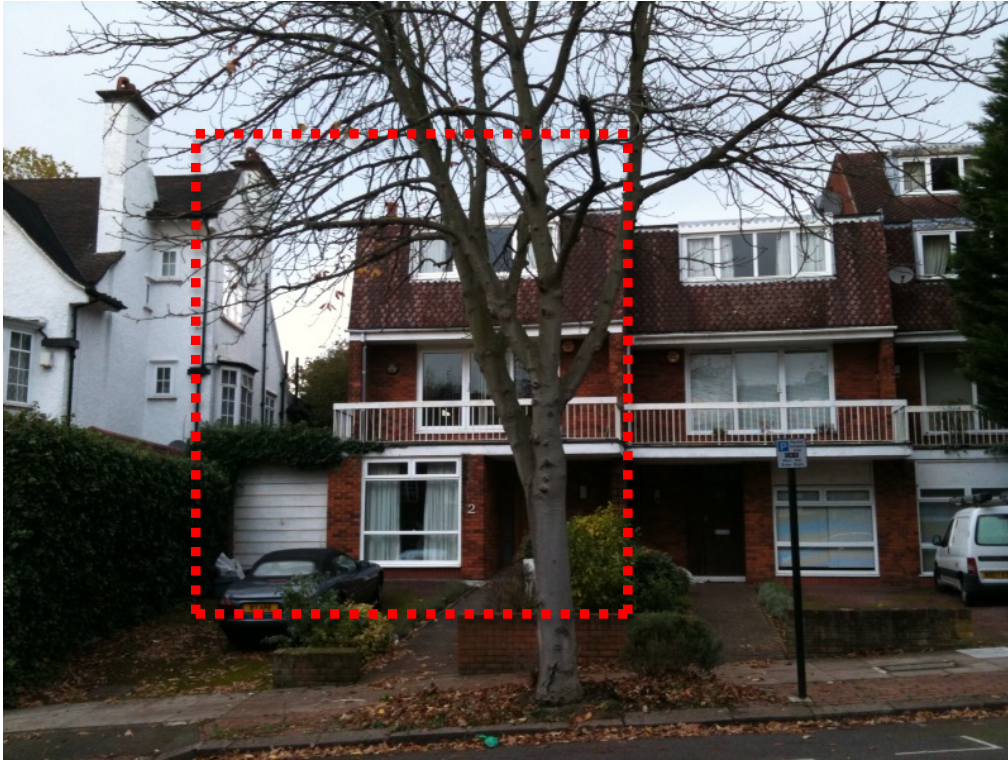
No. 2 Oakhill Avenue which forms the end of terrace.
