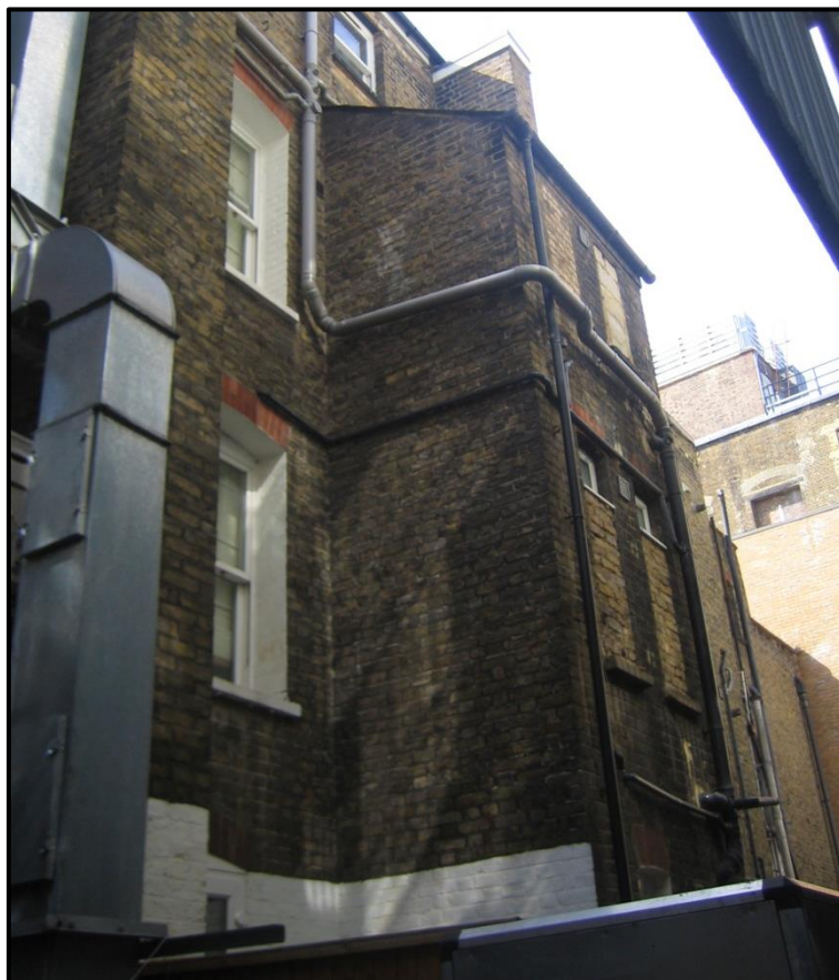
Fig. 3: Existing View: Rear elevation showing the extract system to the neighbouring property
