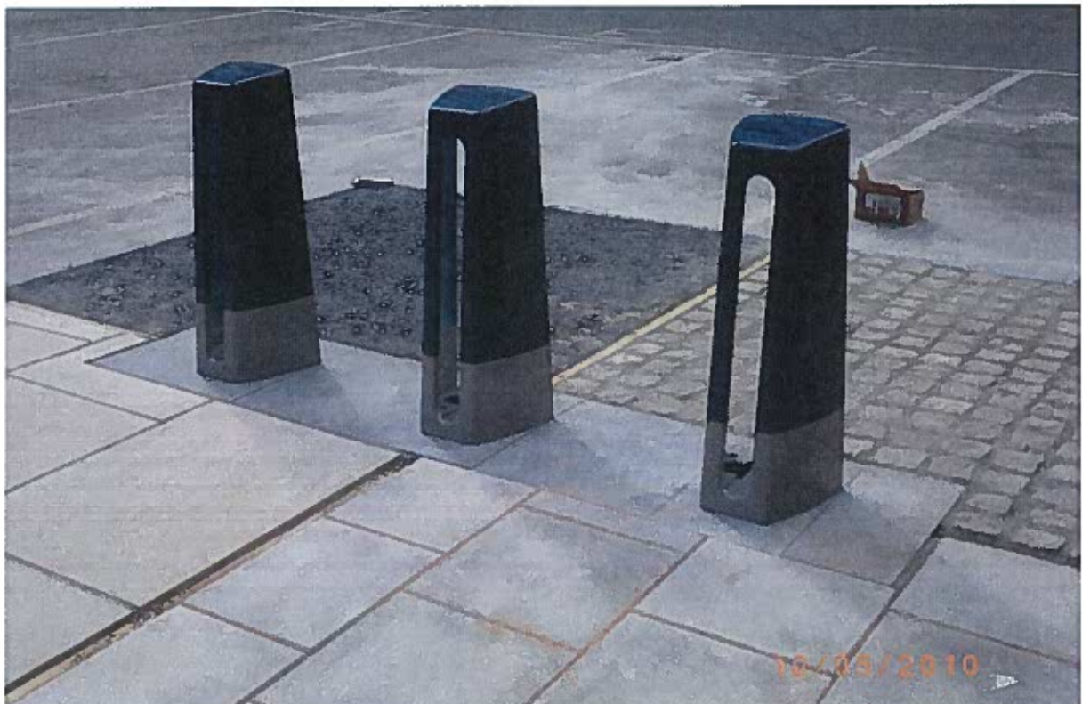
Figure 4: Mock up installation in four different pavement types- clockwise from top: tarmacadam, granite setts, concrete pavers, York stone pavers. Note that the pavements
