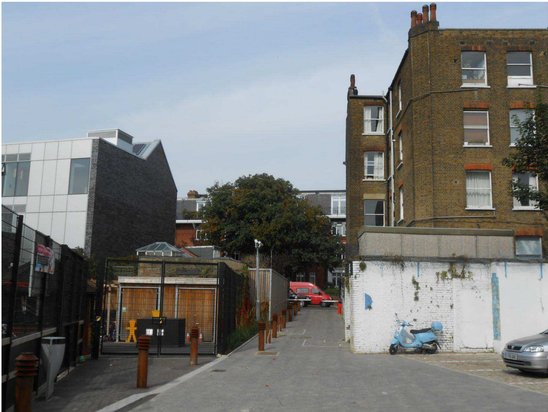
View of rear of site looking North from Mill Lane open space. School playground to left. Cavendish Mansions to right.
