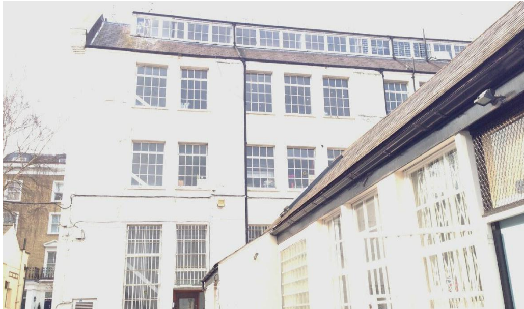
Figure 2 – Rear Elevation to Leeder House
