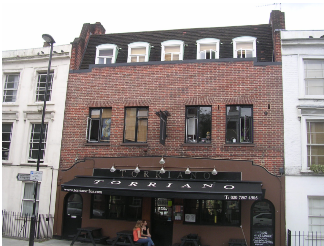
View of the pre-existing Crittall windows at 1 st floor and timber windows and 2 nd floor (from archive)
