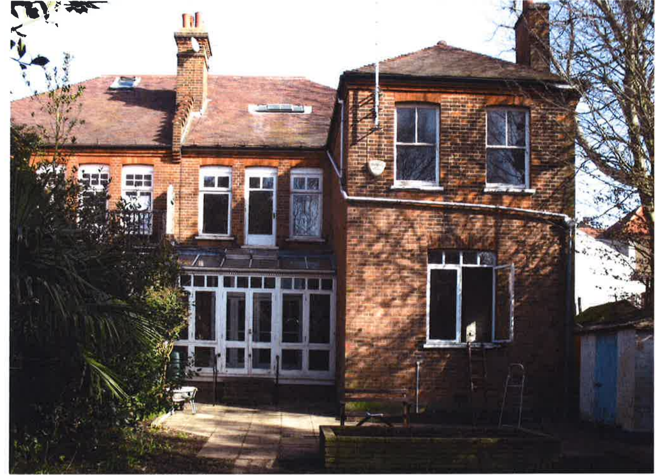
View of Rear Elevation of no. 2 Clorane Gardens
