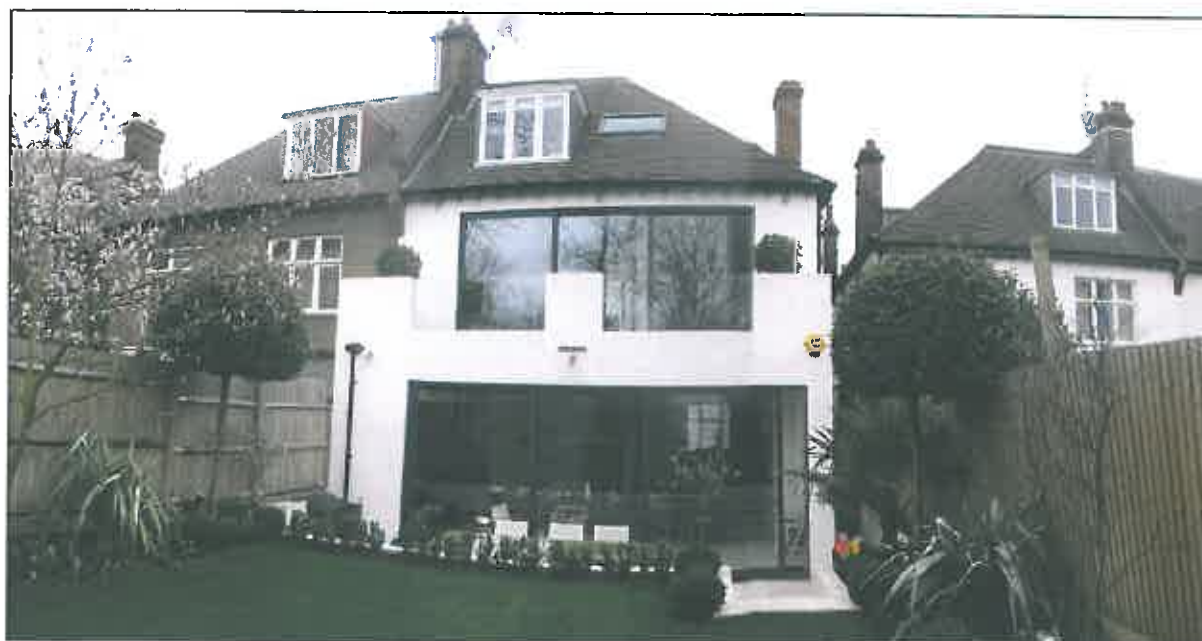
View of 10 Antrim Grove from back garden
