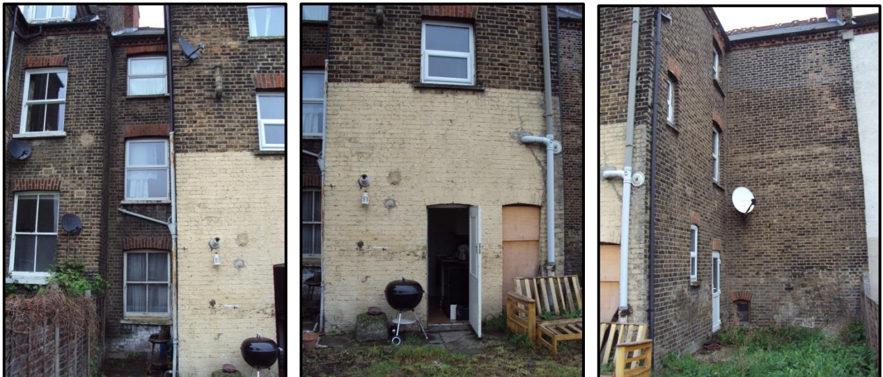
Fig. 2-4: Rear Elevation images of 163 Sumatra Road
