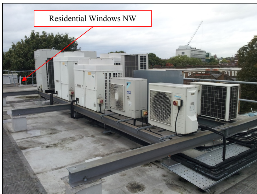
Roof Plant (NW)
