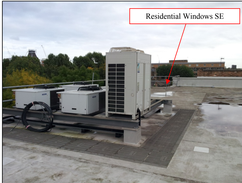
Roof Plant (SE)
