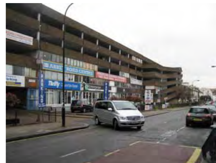
CAR PARK LOOKING EAST
