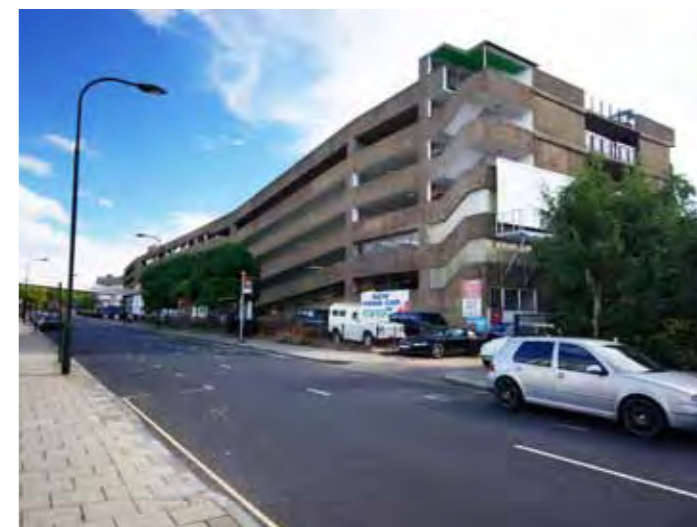
BELSIZE ROAD LOOKING EAST AT EXISTING CAR PARK
