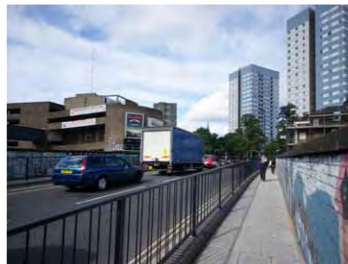
ABBEY ROAD BRIDGE LOOKING NORTH
