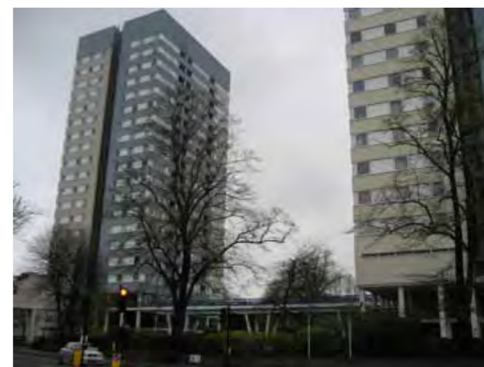
EXISTING TOWER BLOCKS FROM ABBEY ROAD
